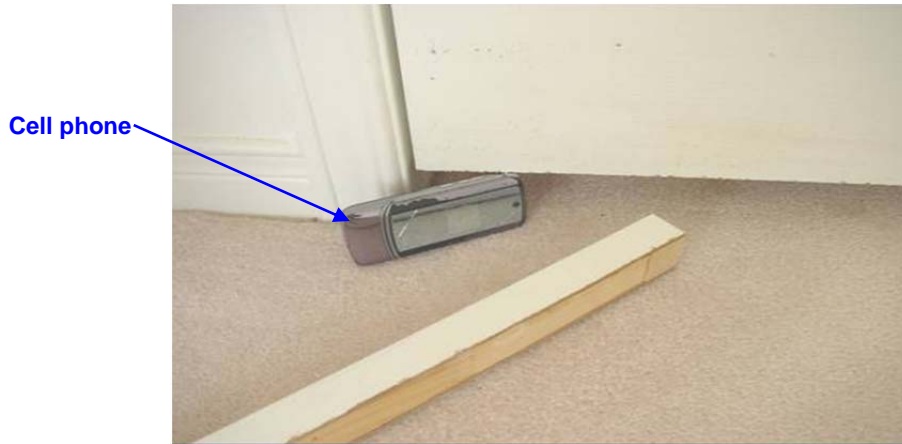
Figure 2: Photograph of Undercut of Bedroom Door
