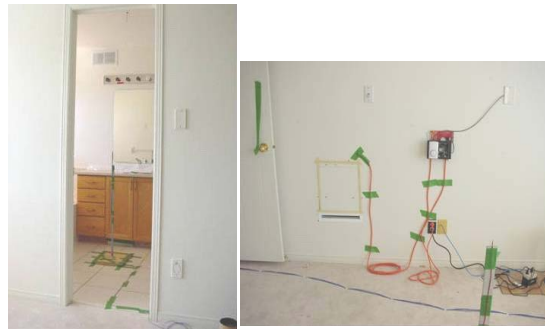
Figure 8: Photographs Showing Location of Air Share and Stud Cavity in Bedroom 2
