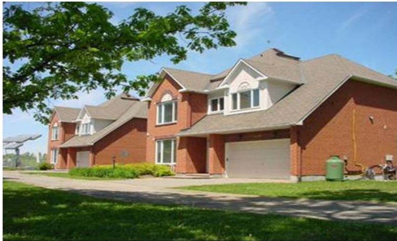
Figure 1: Photograph of Exterior View of Houses Showing Experimental House Propane Tank (May 2011)
