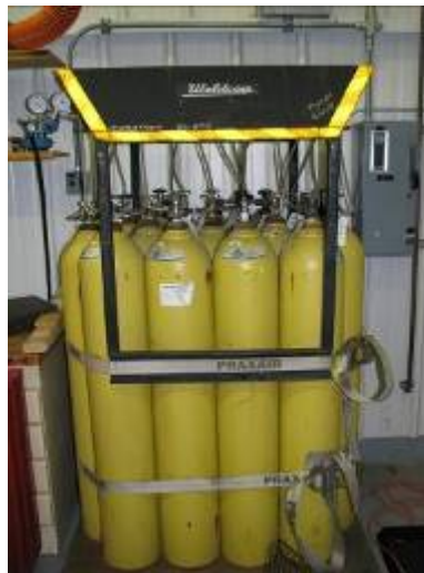
Figure 21. Compressed air tanks for supplemental air supply.
