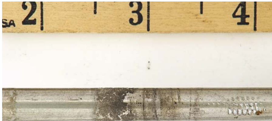
Figure A-61. Higher Magnification View of the Corrosion and the Interaction Region between the Valve Stem and the Guide Washer from PRV 41
