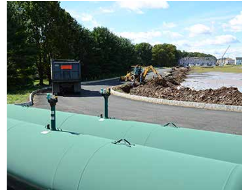
Carriage Hill’s 563 condos, townhomes, and single-family houses are served by an individually metered central propane distribution system.
