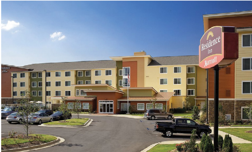
The Residence Inn by Marriott in Florence, Alabama, used a 17-unit gas tankless water heater array to save space in the mechanical room and allow room to service the units.
