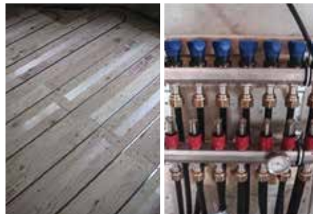
Examples of in-floor hydronic radiant tubing (left) and a distribution manifold (right).
